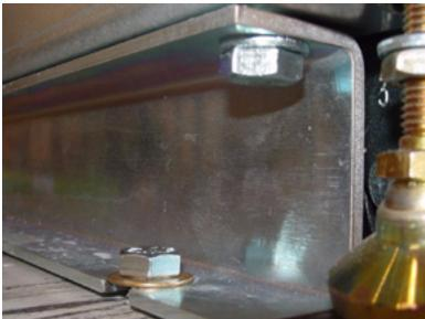
12. Check the bubble level on the floor of the cabinet on the right hand side of the Power Conversion Module (see **Figure 24**). The Liebert FS is sufficiently level when the bubble is within the outer of the two circles. If the bubble is outside the outer circle, use the leveling feet to adjust until bubble is within the outer circle.
